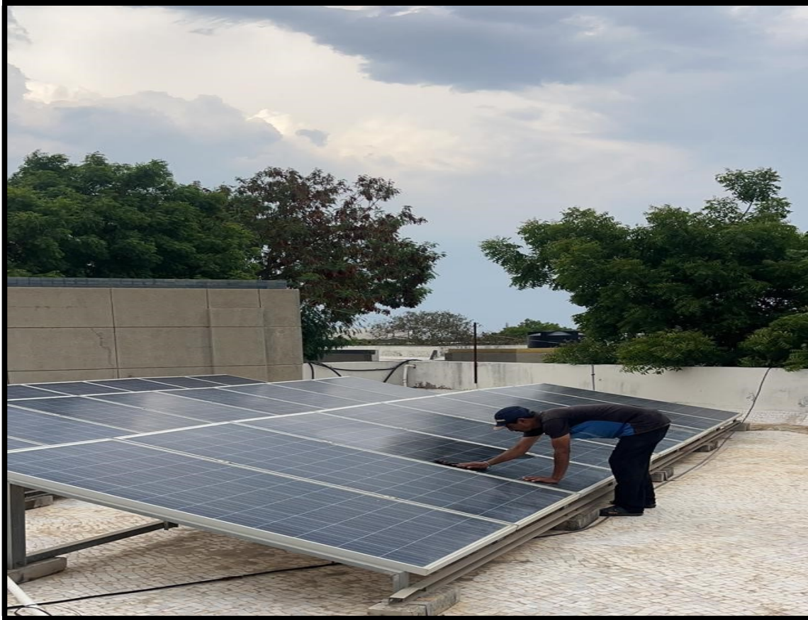
HEAT ISLAND EFFECT ROOF--CHINA MOSAIC ON ROOF TOP
